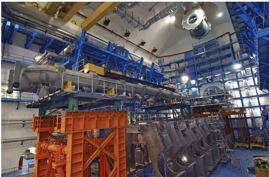
Figure 9.13: Lowering of the barrel LAr calorimeter down to the cavern in October 2004. The first barrel toroid coil can also be seen on a temporary support platform before it is installed in the cradles of the feet.
